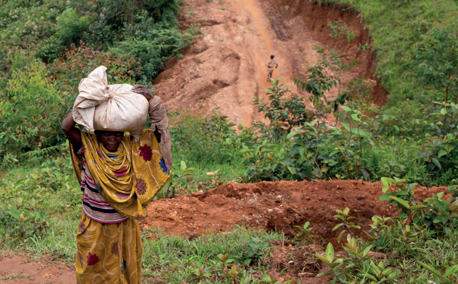
Villagers carry rocks and sand up the hill in Gisheke, where a new community is being built after many of residents lost their homes in landslides.
